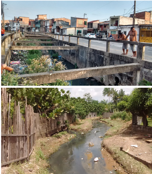
Figure 6 - Examples of sewage in Belém and Macapá
